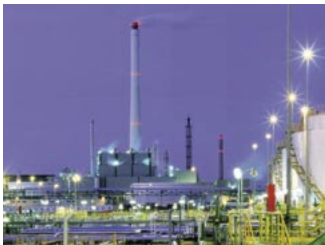
1 Kraftwerk STEAG Leuna 1 Power plant of STEAG Leuna
